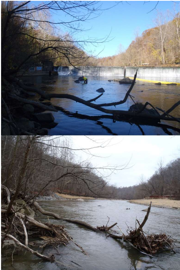
Figure 5-4: Simkins dam on the Patapsco River, before and after its removal in 2011
